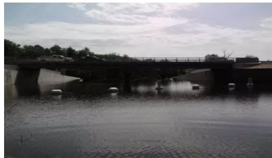
Spillway Upgrade Project
