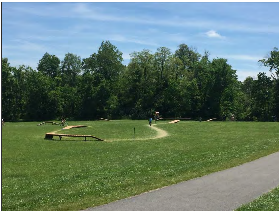
The Bike Park installed in 2020 along Warrior Drive at Sherando Park
