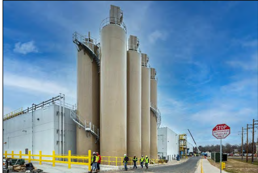
Trex: Second Frederick Co. Manufacturing Facility
