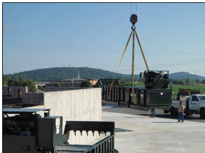
New trash compactor is set in place at the relocated Albin neighborhood citizens convenience site
