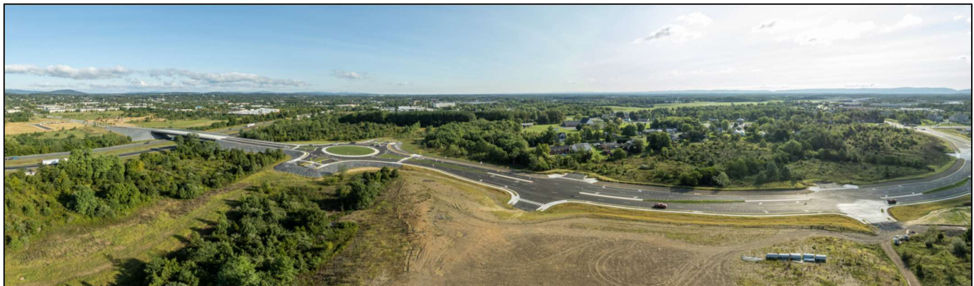
This photo depicts the recently completed Crossover Boulevard. Design and construction of this roadway was managed by Frederick County Public Works. This project consisted of a 1.07-mile road including a 321-foot bridge over interstate 81 and a two-lane round-a-bout connecting future Warrior Drive. This project was completed on-time and under budget and serves as a much-needed arterial connector between eastern Frederick County and the City of Winchester. Public Works is currently working through the design phase of its next transportation project: Renaissance Drive located in the Kernstown area.
