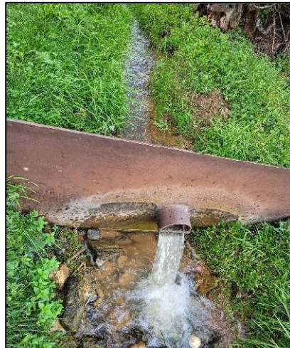
Point where the leak is measured
