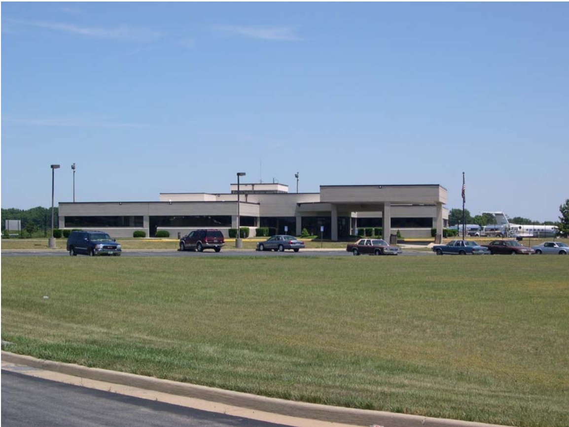
Winchester Regional Airport Winchester, Virginia Established 1987
