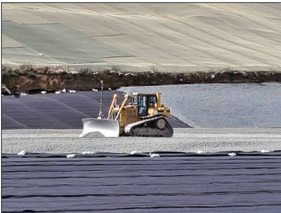
Contractor is nearing final completion of MSW Cell 3A, an eleven acre area that is being prepared for future placement of solid waste. This photo shows a dozer placing the one foot layer of leachate collection stone in the bottom of the new cell.
