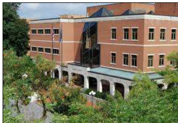
Winchester-Frederick County Joint Judicial Center
