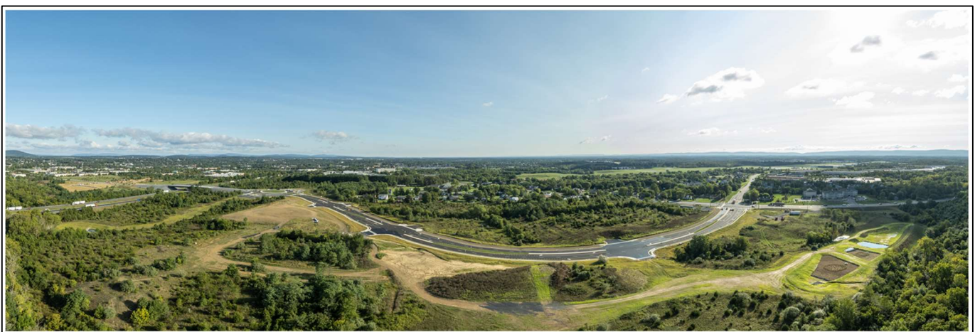
Crossover Boulevard at project completion September 2021. $22 million Dollar Public Private Partnership.
