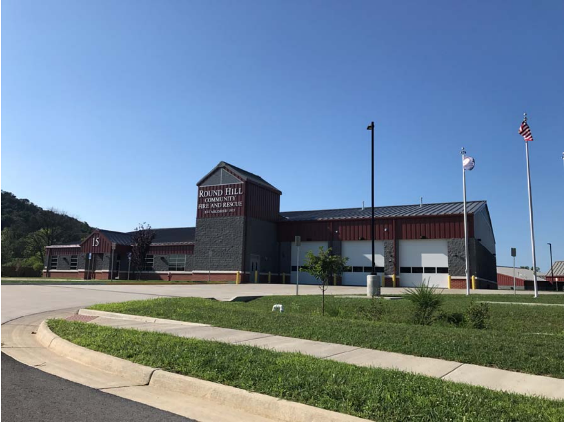
Round Hill Station Frederick County Fire and Rescue Winchester, Virginia Opened August 2015
