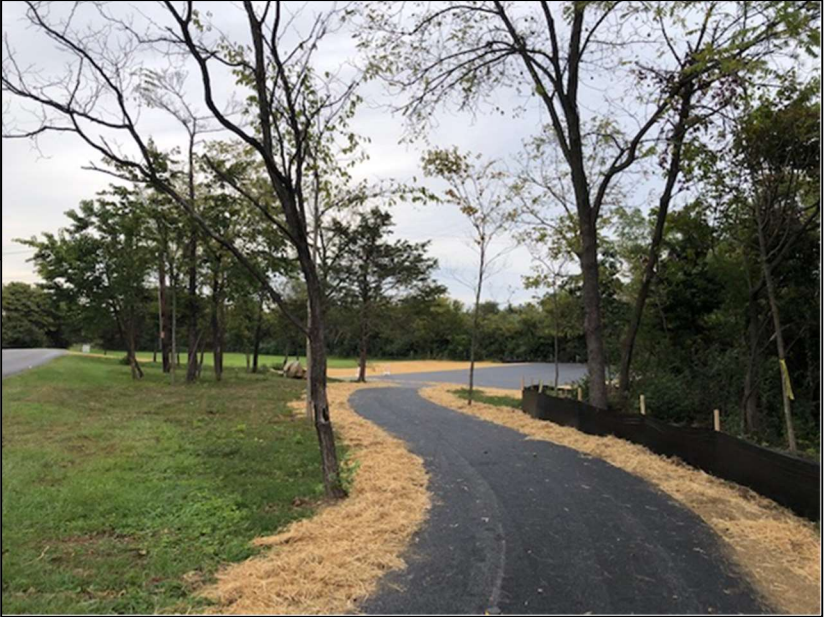
Newly installed path at Clearbrook Park
