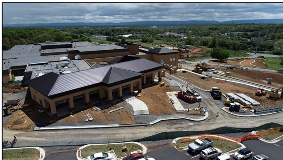
James Wood High School addition and renovation project
