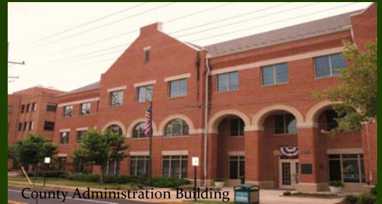
County Administration Building
