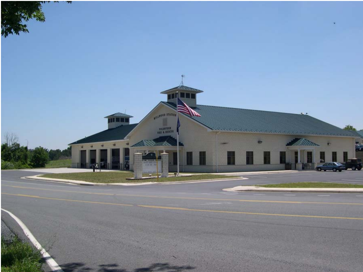
Millwood Station Frederick County Fire and Rescue Winchester, Virginia
