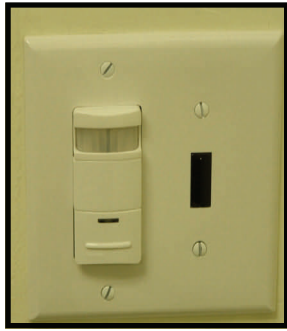
Automatic light sensors were strategically placed throughout County buildings.
