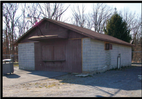
Old Concession/Restroom at the beginning of renovation work.
