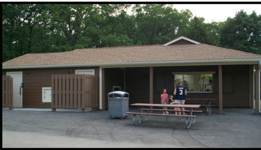
The new building-on time and under budget.....procurement at work.
