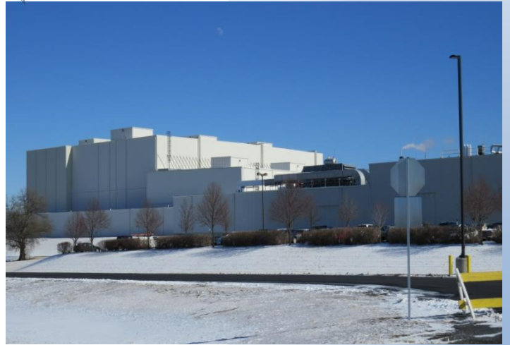
HP Hood Dairy Addition
